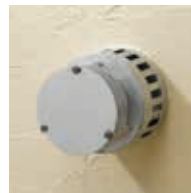
Balanced Flue (No chimney required)
